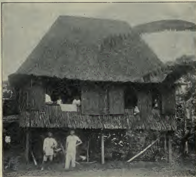
FIG. 333. — A house in the Philippines, built of bamboo and covered with thatch. The house is raised above the ground because of the dampness.
